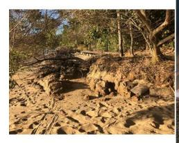
Erosion scarp with geobags placed to prevent further erosion
